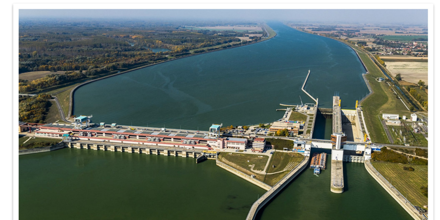
Gabčíkovo power plant
